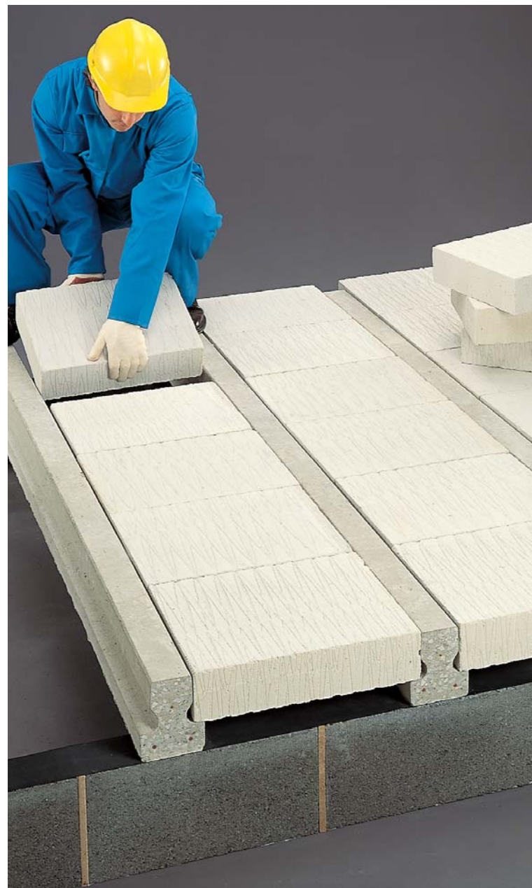
The blocks provide a strong and firm floor base.
