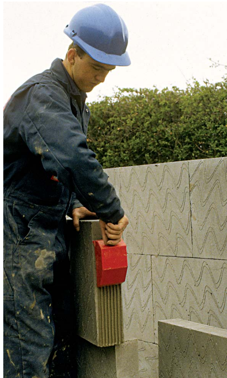
The pre-mixed mortar is easily applied and Aircrete blocks, manufactured to such a high degree of dimensional accuracy are ideal for use with thin joint mortars.
