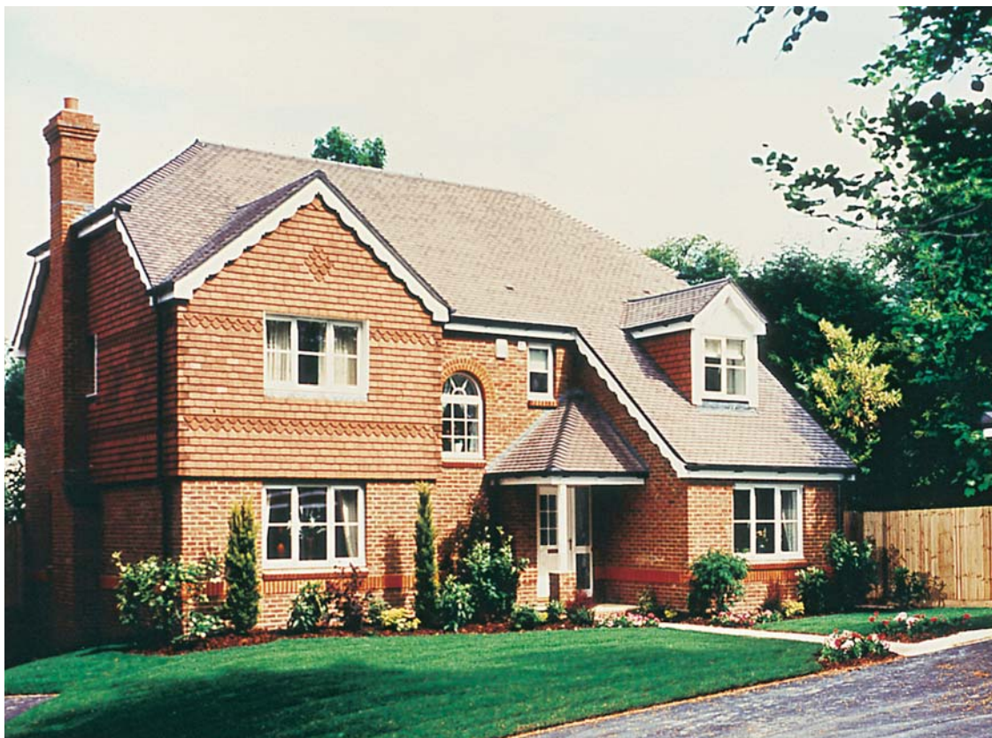
The adoption of the thin joint technique has allowed leading housebuilder CALA Homes to radically shorten its build times.
