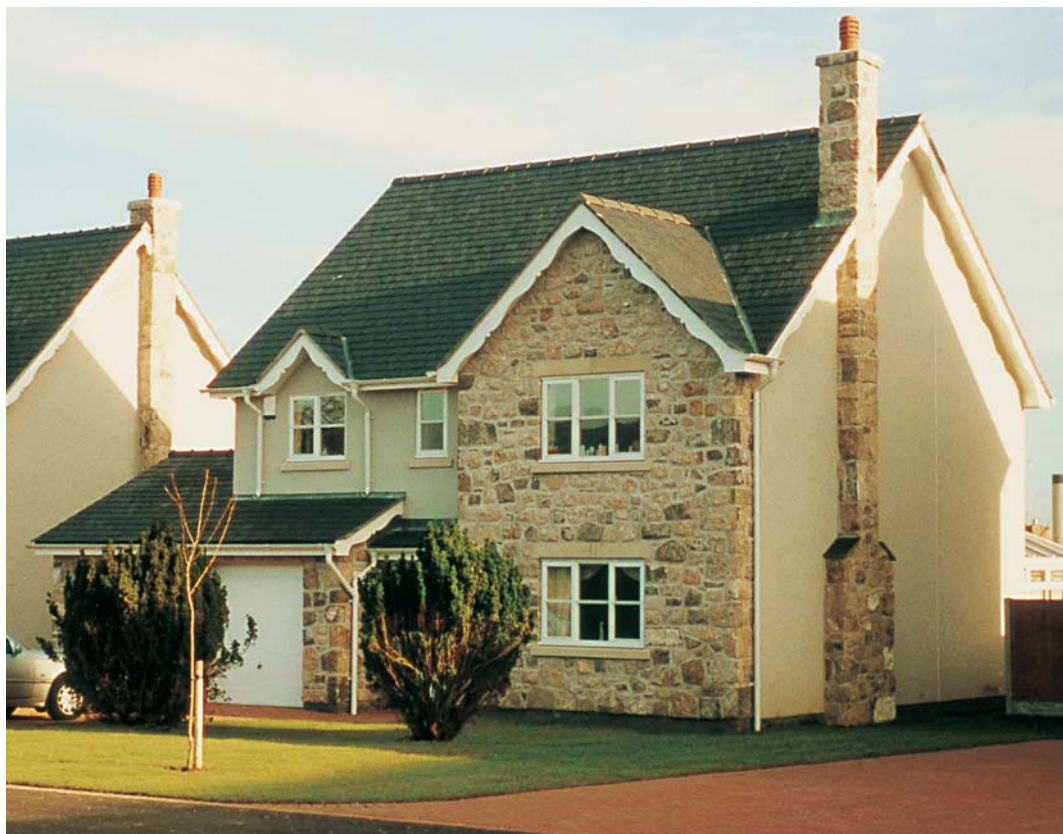
Due to an inherent combination of strength and insulation, Aircrete solid wall construction is the method favoured by housebuilders Newhaus Systems.
