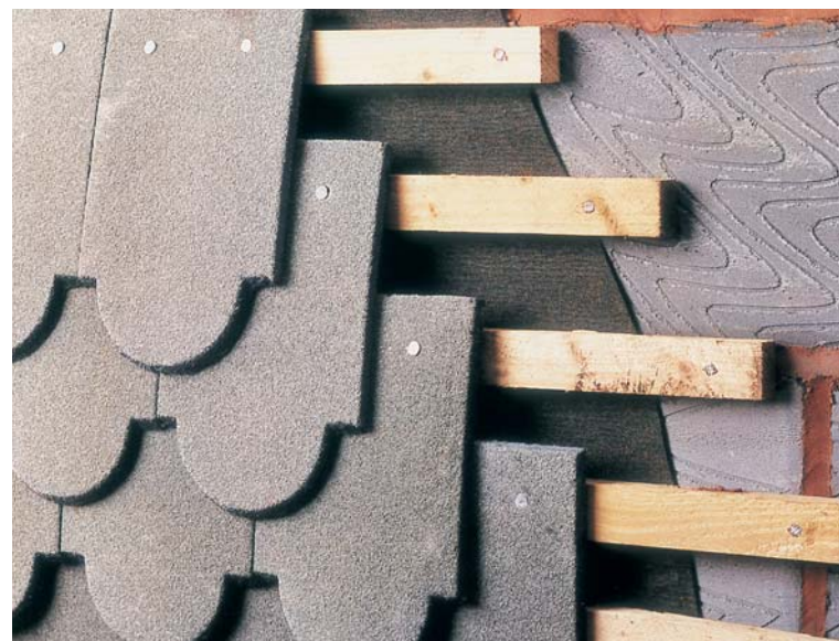
Such is the versatility of Aircrete that it permits a wide range of finishing options. Tiles can be secured onto timber battens and positioned directly onto the blockwork to produce an elegant façade.
