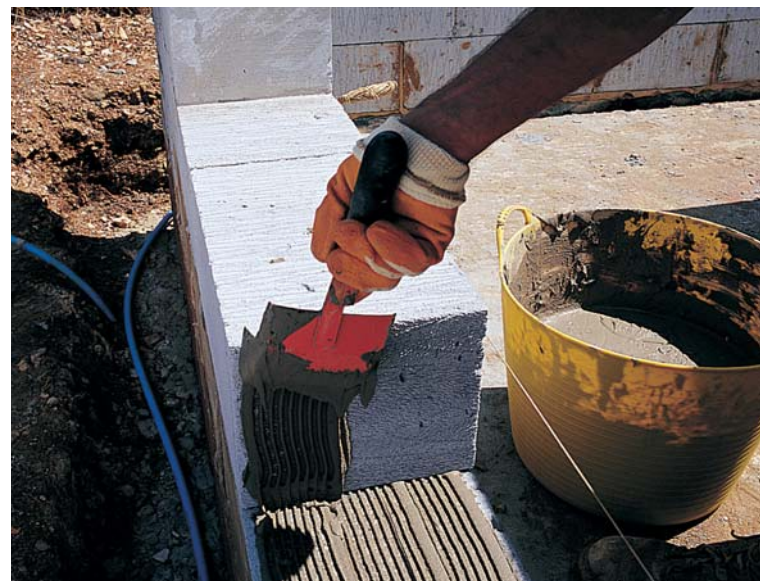
Aircrete's ease of handling and lack of cavity enables a rapid build to eaves level, allowing the roof to be completed earlier. Finishing trades can commence sooner, resulting in a significant reduction to the overall completion time.
