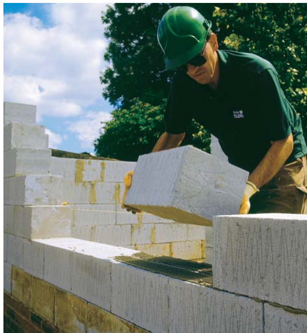
Aircrete is an inherently safe building material, and indeed offers many health and safety advantages over other materials.
